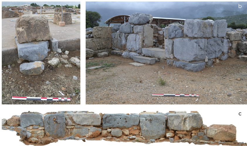
Fig. 7 Ironstone building components of the lower elevation of the Protopalatial West Façade reused in the Quartier d'apparat (a; K. Papachrysanthou), the Dungeon (b; K. Papachrysanthou) and the South Façade (c; G. Cantoro) of the Neopalatial Palace. © EFA.
